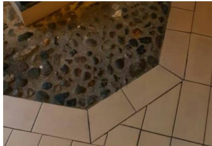
Figure 3.3(d) : Image of pebble stones indoor drainage (Lim,2017)
